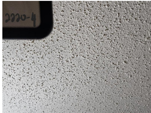
2220-4 Surfacing Texture (3% Chrysotile) Typical Interior Walls/Ceilings
