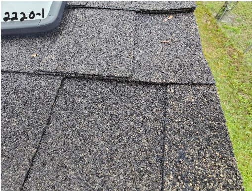
2220-1 Asphalt Shingle/Tar Typical Exterior Roof
