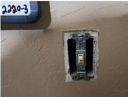
2220-3 Joint Compound (2% Chrysotile) Drywall Typical Interior Walls/Ceilings
